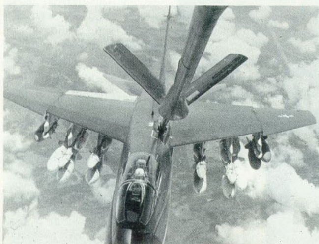
The sixth Air Force A-7D (AF68-8220) took part in Project Seek Eagle, at Eglin AFB, near Valparaiso, Florida (Hq. of Air Proving Ground Centre and Tactical Air Warfare Centre) and is seen here with four pylons supporting 20 \times Snakeye Mk. 80 retarded-fall bombs each weighing more than 300 pounds. Painted stripes are for telemetering only. The Navy arrester-hook is retained on all A-7Ds. (Below) Third A-7D (AF67-14584) flown by John D. Konrad, undergoing Boeing KC-135 simulated in-flight refuelling development tests. Bomb clusters add up to 12,500 pounds. (Photos: US Air Force via Vought)
